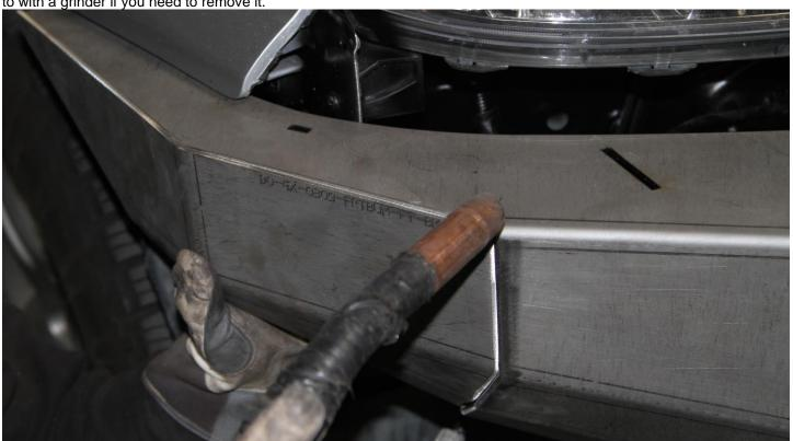
Step 12.) you can now take the DS and PS filler 1 plates and attach them as shown in the picture. Make sure all your edges are ground down with a soft wheel grinder at a 45\* angle for the best welds and strongest welds.
