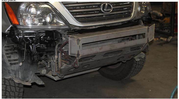
Step. 8) At this point once it's Tacked together you can jump over to the installation instructions for the 03-09 of the GX bumper (step # 18) and we highly recommend you test fit the bumper onto your GX before you go any further.
